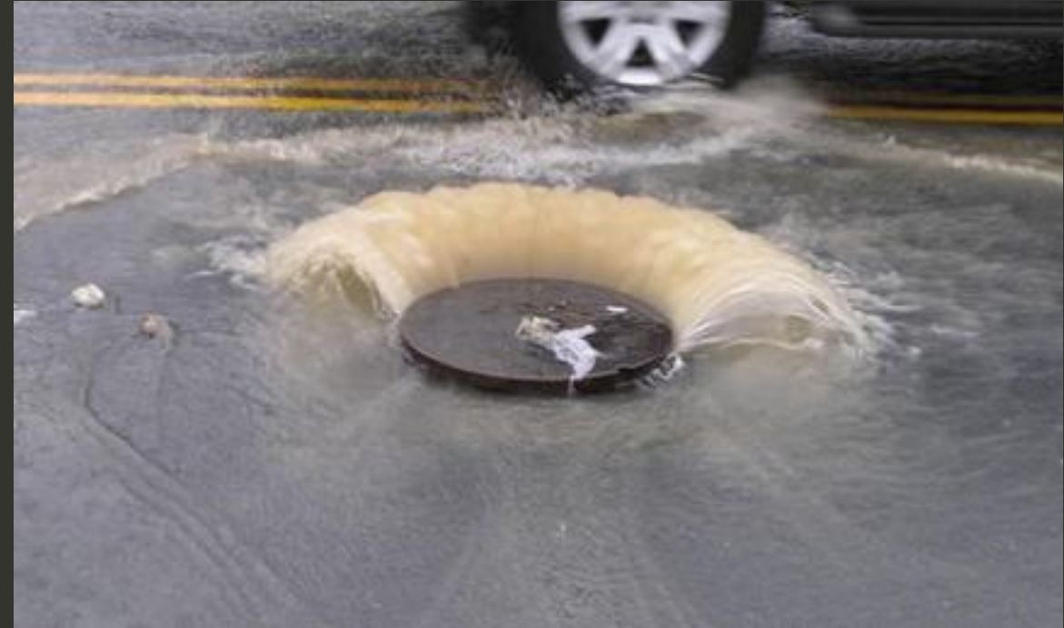
Combined sanitary sewer overflow / WPR
